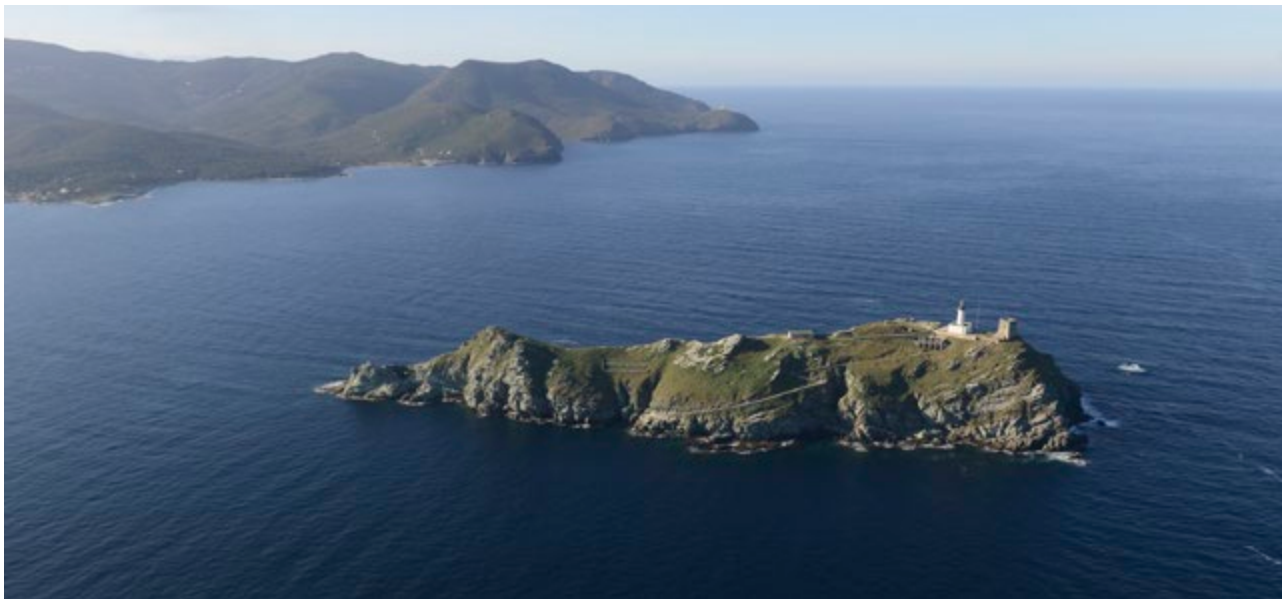
Figure 1. The Giraglia island seen from the North-East. © F. Rombaldi/assoc. Finocchiarola.
