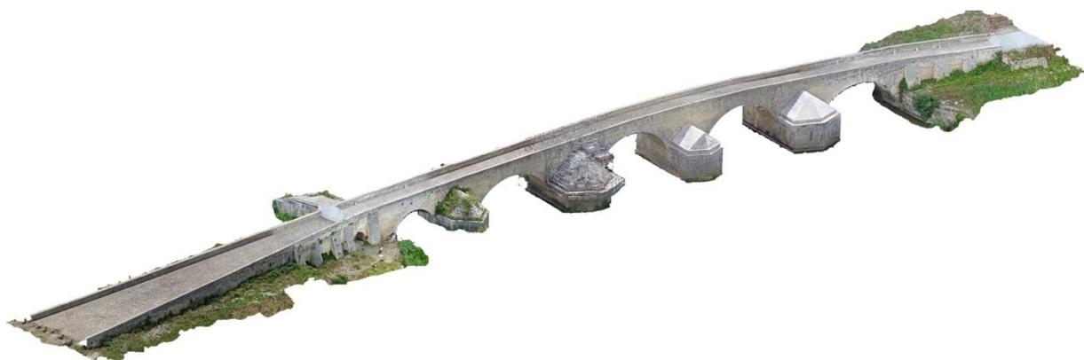
Figure 6. Axonometric view of the bridge elaborated using drone technology and aerial photogrammetry.
