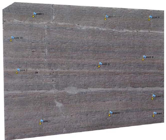
Figure 6. Numerical model (point clouds) of the letter of Harkhuf preserved on the main façade. The flags show the Ground Control Points (GCPs) necessary to scale the model. The letter contain 60 million of points.
