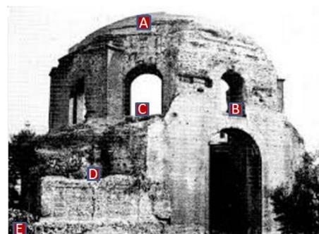
Figure 8. Ambient vibration measurement points on the main façade of the monument (view from North).
