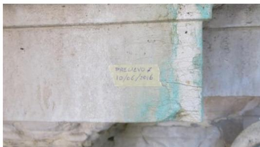
Figure 1. Neptune's Fountain of Giambologna – Bologna, Italy; a portion of stone material stained in a light blue color. The stains are caused by the percolation of the corrosion products of the overlying bronze elements.
