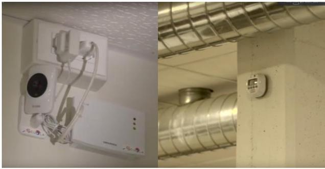
Figure 6. Examples of the installed sensors in the building spaces: sensor of presence and sensor of temperature and humidity.
