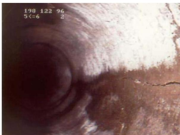
Figure 3. Inspection image showing fissure [14].
