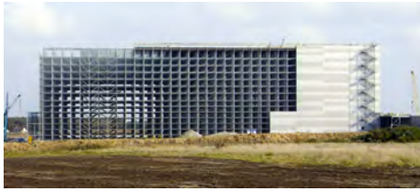
FIGURE 4. Example of a warehouse building under construction (Google Maps [2]).
