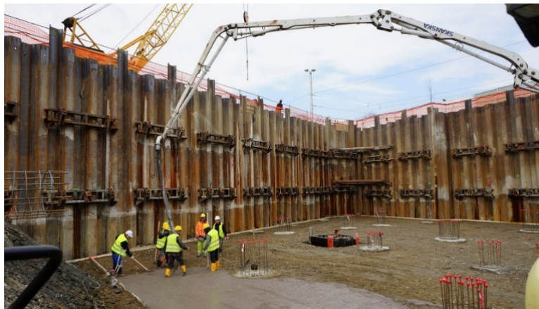
FIGURE 5. The first ready mix concrete placement.
