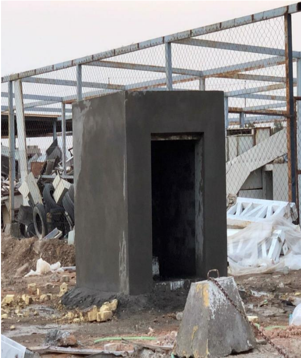
Figure 3. Covering the walls with cement mortar.
