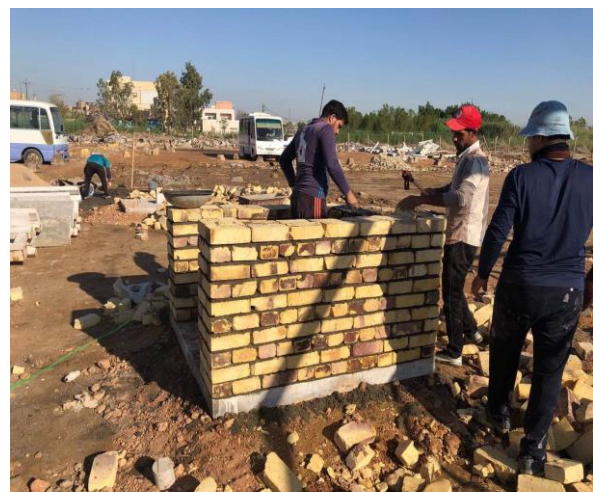
Figure 2. The construction process of the structure (walls).
