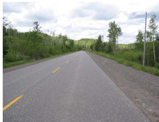
Figure 1. Daytime view, looking north, of the 800 m section of Highway 527, approximately 20 km northwest of Thunder Bay, Ontario, Canada, used in determinations of moose detection distances on a highway at night.
