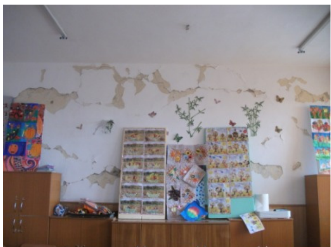
Figure 6. Cracks in the school walls in Focșani (source: the Vrancea newspaper; http://www.ziaruldevrancea.ro ).
