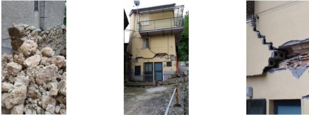
Figure 5: a) Travertine blocks of a collapsed building, b) Building with two added floors made of hollow bricks, c) Detail of the hollow
