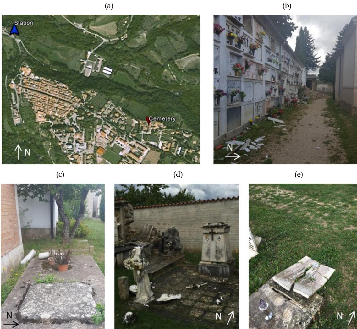
*Figure 1. Location of the cemetery and of the seismic station at Amatrice (a), damages to statues, monuments and graves in the Amatrice cemetery (b-e).*
