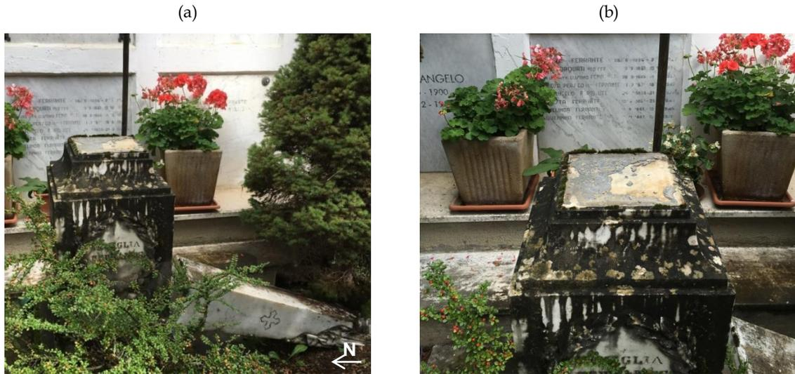
Figure 2. Damaged obelisk in the Amatrice cemetery (a), particular of the base section (b).
