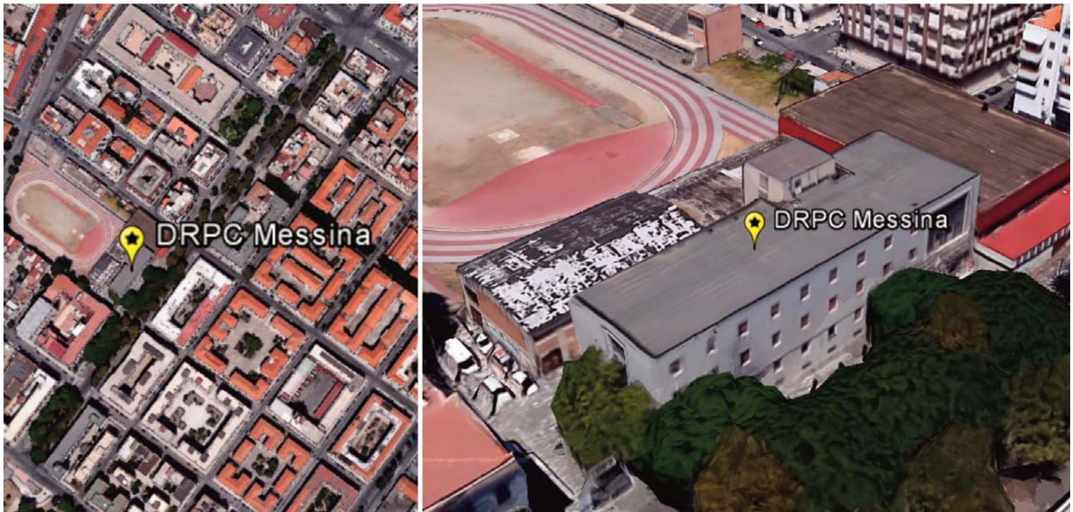
FIGURE 2. INGV - DRPC - Messina Building.
