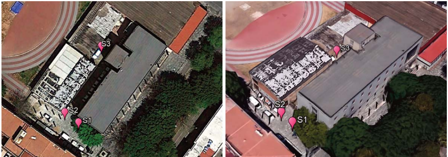
FIGURE 9. DRPC - Messina building.
