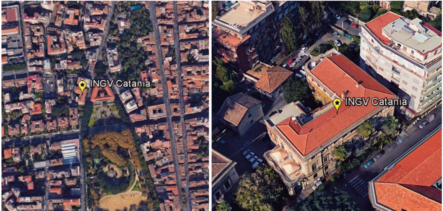
FIGURE 1. INGV - Catania building.
