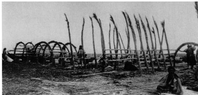
Figure 2 : Construction of reed houses
