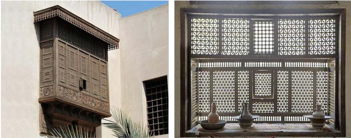
Figure 1. Example of a Mashrabiya in exterior shot (on the left) and in interior shot (on the right)
