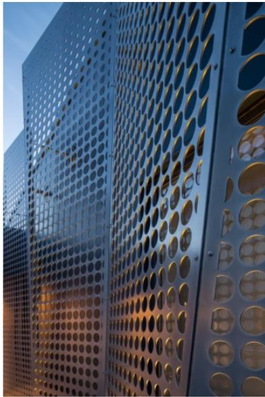
Fig 10(c) Screening of perforated metal sheet with circular shapes (dezeen.com)
