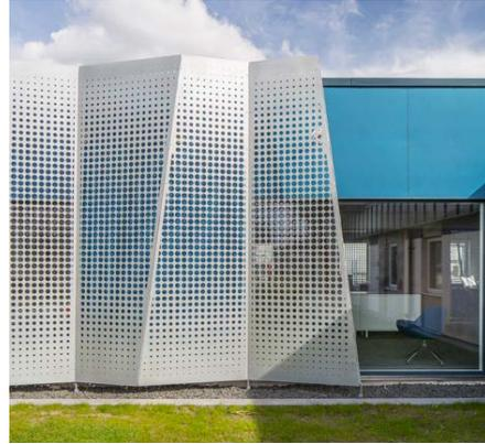
Fig 10(b) Screening of simple punched metal sheet
