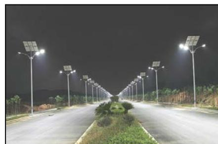
Figure 10a – Live Solar LED Street Lamps
