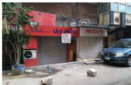
Figure 11. Sidewalks distortions in terms of widths, paving, regularity, and levels (The researcher, 2017)
