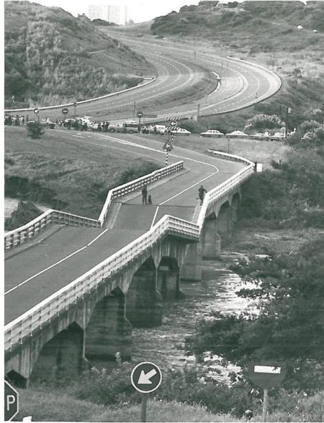
Figure 3. Caissons failure due to bed erosion (Frankipile, 2008)
