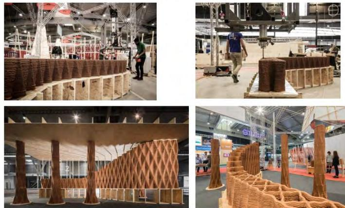
Figure 15. Robotos driven by cables & drones have helped in 3D printing using clay in printing large scale construction
