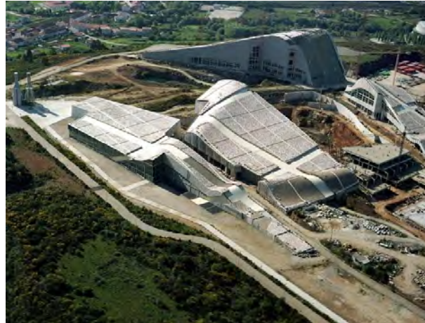
Figure 9. The City of Culture. Architect: Peter Eisenman
