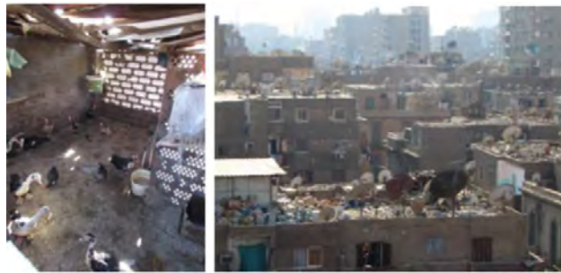
Figure 1. Poultry room with red brick; Neglected rooftops in downtown Cairo. Source: https://webpages.uidaho.edu/larc380/new380/pages/greenRoof.html
