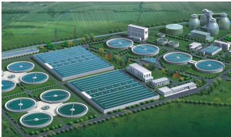
Figure 1: The main structure of sewage treatment plant in Enterprises
