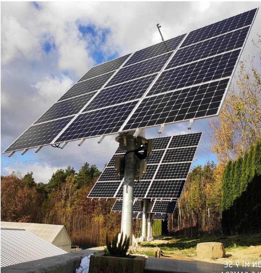
Figure 2: Sun-tracking modules of PVT panels (original image from the RESHeat project demo sites)
