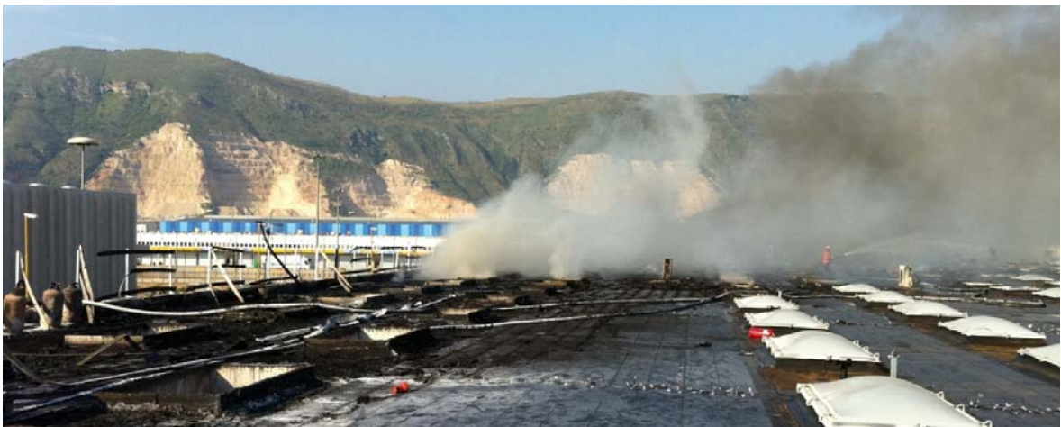
Figure 5: A large warehouse involved by a fire, probably external at the PV plant but strongly influenced in his growth and propagation by the photovoltaic layers.
