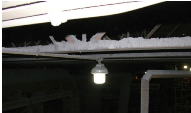
Figure 2: Iron dust deposits on elevated surfaces at Hoeganaes Corporation facility (CSB, 2011).
