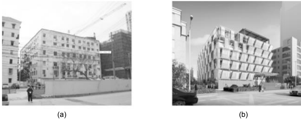
Figure 1: Comparison of building exterior before and after reconstruction
