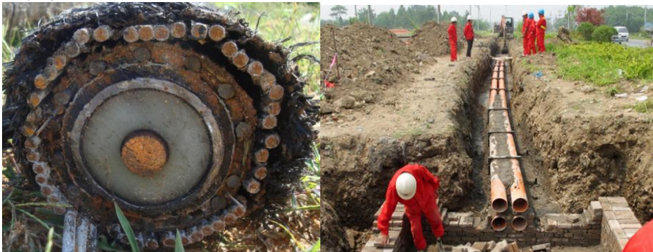
Figure 5: The photos of cable lines and FBG sensors installing and burying
