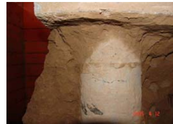
(a) The lateral crack of the pile cap (b) the distribution map of cracks (c) Pile 2# cracking and soil separating
