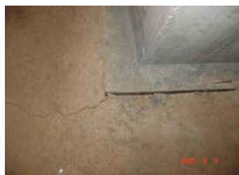
(a) The lateral crack of the pile cap (b) the distribution map of cracks (c) Pile 2# cracking and soil separating
