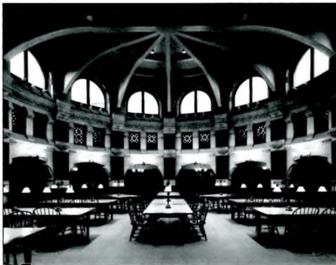
In the rotunda reading room in the newly restored Furness Building at the University of Pennsylvania, the exposed iron beams that support the roof curve down to meet delicate terra cotta floral ornaments that top the sturdy brick pilasters. Photo credit: Dardas.
