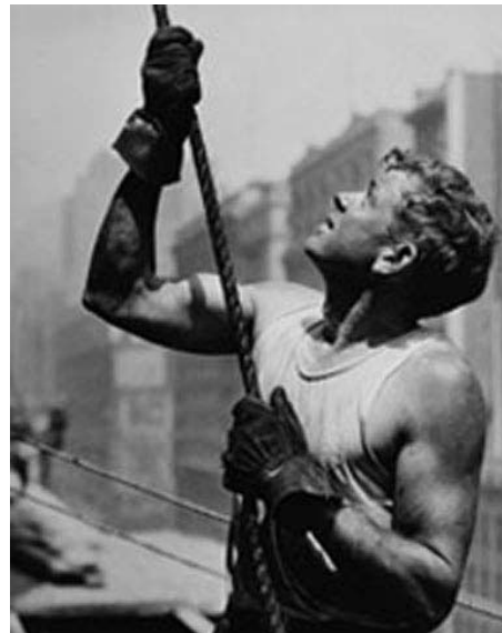
"Steady! Construction of the Empire State Building, 1930-1931". Gelatin silver print by Lewis Wickes Hine. From a series of photographic documents of social conditions, 1905-1939. Photography Collection, Miriam and Ira D. Wallach Division of Art, Prints, and Photographs, Humanities and Social Sciences Library, The New York Public Library. Used with permission.
