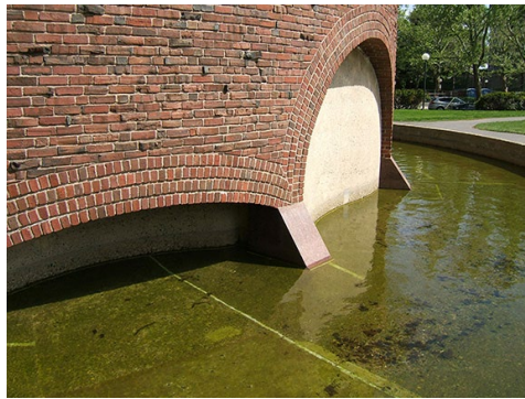
Figure 10 - Light wells from exterior (Kresge Chapel)
