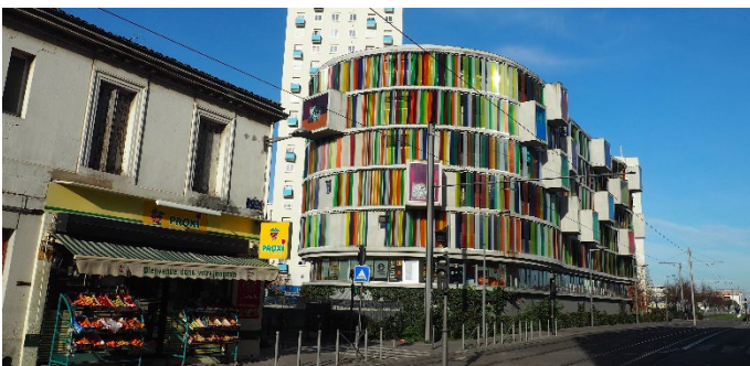
Fig. 7. Arc-en-Ciel building. Photo © A. Herbert.
