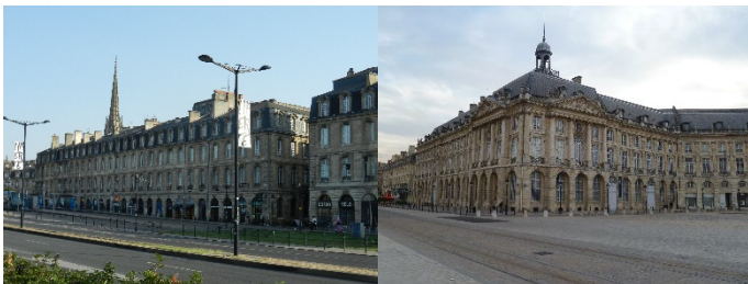
Fig. 2. Bordeaux, city of stone. Photos © A. Herbert.
