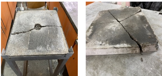
Fig. 4. Typical failure behavior of unreinforced concrete slabs.
