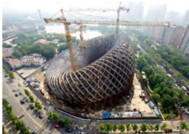
Figure 16. Phoenix InternationalMedia Center. Source ("Phoenix International Media Center", 2011)
