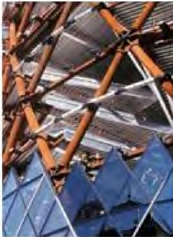
Figure 13. (Swiss Re Headquarters) under construction
