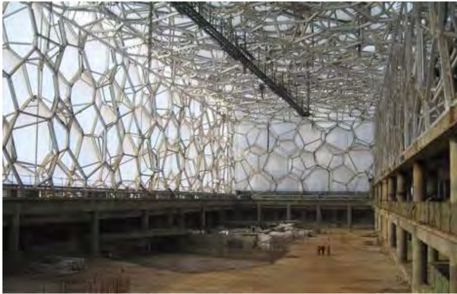
Figure 11. Watercube National Swimming Centre structure system, interior.
