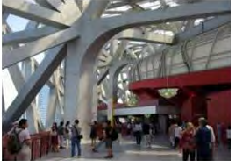
Figure 12. Bird'sNest Stadium n China, exterior.
