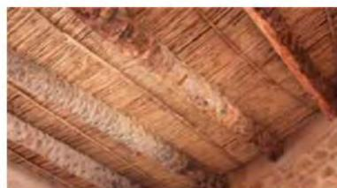
Figure 3. Palm Trunk Beams used for traditional roofing in Sinai (Ibrahim, 2010)
