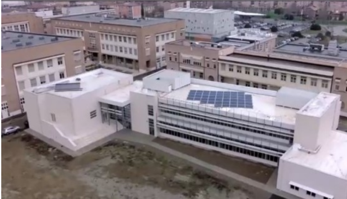
Figure 1. Flatroof with cool white waterproofing membrane (Tecnopolo building of the University of Modena and Reggio Emilia, Modena, Italy).
