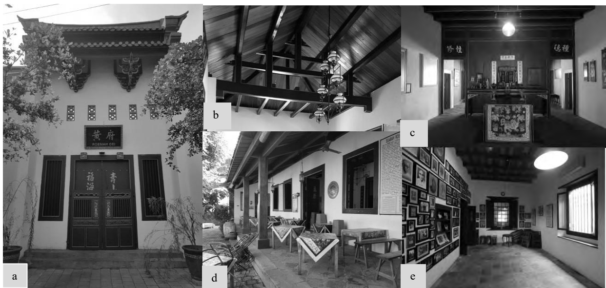
Figure 4. The original main building of the Oei House: (a) the main gate, (b) the exposed roof construction frame, (c) the main hall in the main building, (d) the front terrace functions as a café, and (e) the Oei family museum
