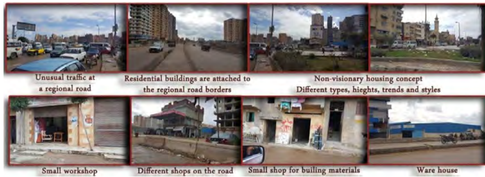
Figure 6. Facilities at the 45th Road (Yoseph, 2017)
