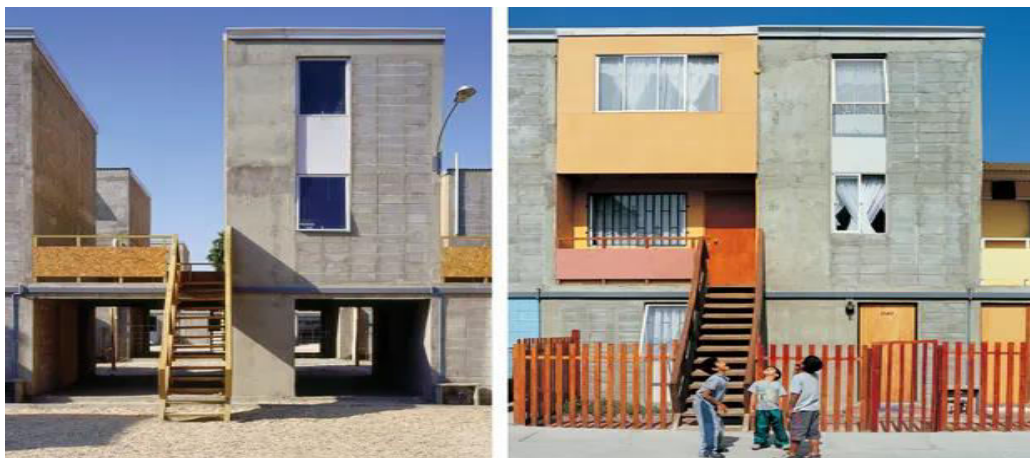
Figure 4: Occupant infill construction at Iquique. Theguardian.com, 2016.
