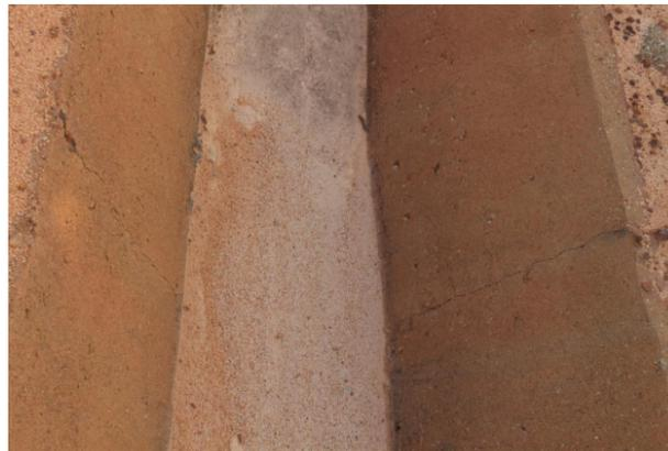
Figure 20: Crack on drainage networks facility, made up from thin plain concrete cross section.
