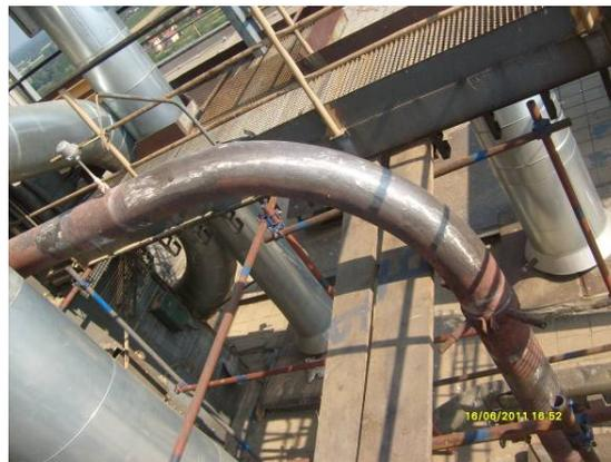
Figure 1: Part of the steam line during NDT.
