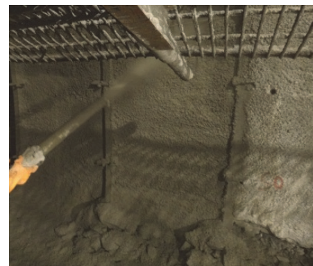
Figure 15: New field shotcrete technology.
