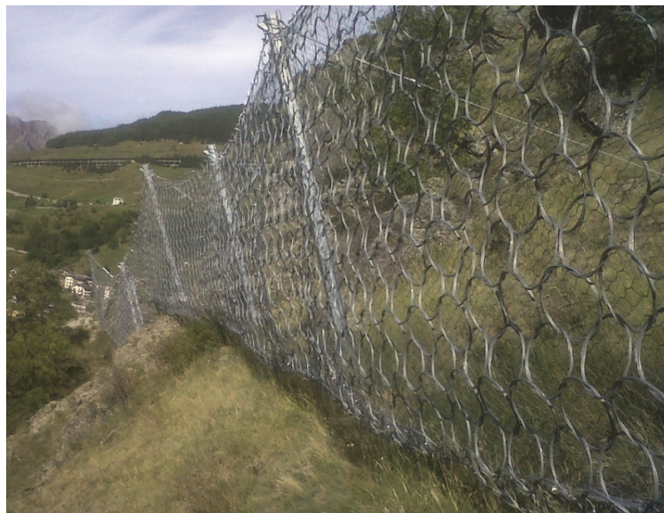
Figure 1: Photo of the studied rockfall protection net fence.
