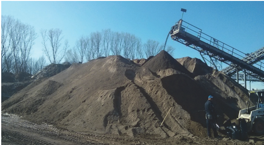
Figure 1: CDW waste treatment plant, Cavit S.p.A., La Loggia- Turin.
