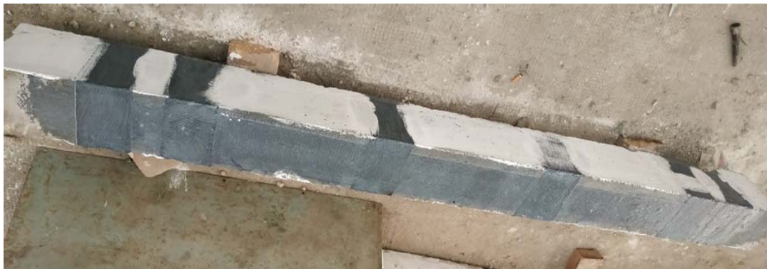
Figure 3: beam after the installation of CFRP.
