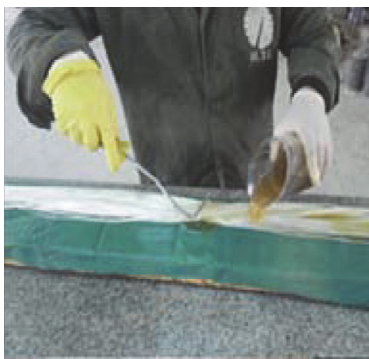
c) Saturating the fibers with the resin.
