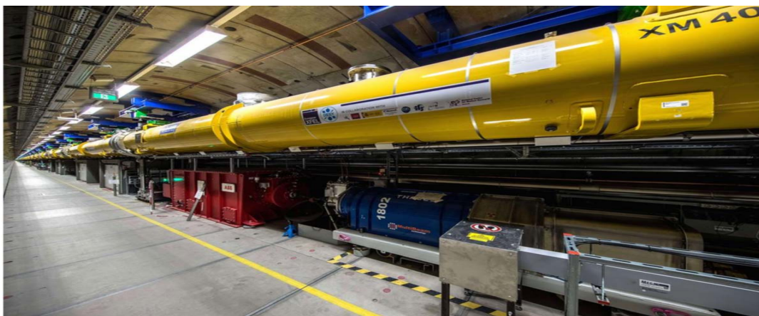
Figure (1): The installation of a train using superconductivity technology
